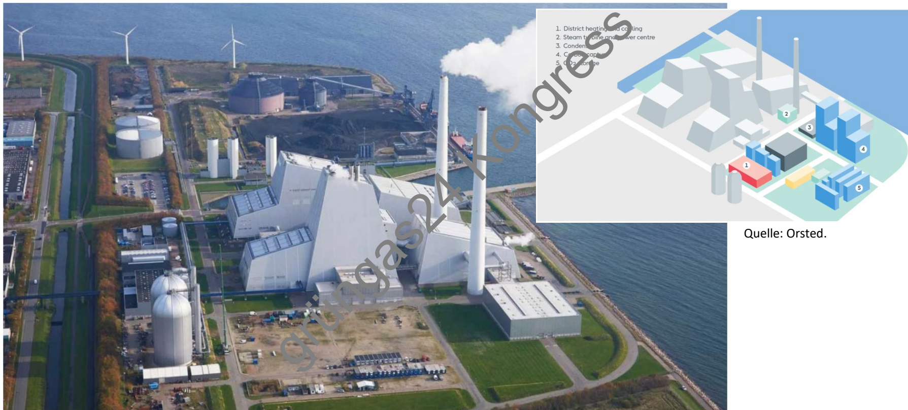
Ørsted's Avedøre Power Station in the Greater Copenhagen area. Credit: Ørsted.
